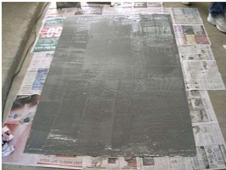
Taking the grout spreader, spread the epoxy out to evenly cover the steel. For more details on the
