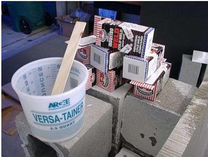
Take a break and heat a bowl of water large enough to hold 16 tubes of JB-Weld. I don't have an exact temperature to give you but you should make the water hot but not boiling. Heating the epoxy will make emptying the tubes, mixing and spreading it much easier and doesn't shorten the pot life enough to be a concern. Let the epoxy soak while you finish prepping the steel.
